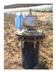
Figure 10 Emergency Gas Relief Vent
