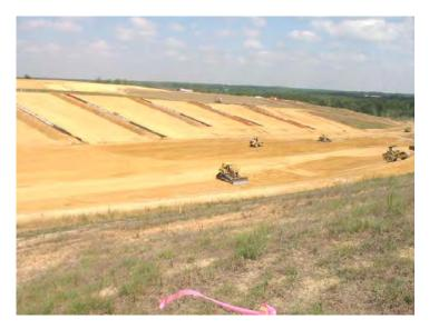
Figure 7 LFG Collector Trenches Installed in Surface of Existing Waste in Piggyback Landfill Application
