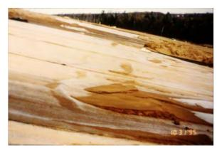
Figure 4 Sliding of Geomembrane and Sand Drainage Layer During Construction
